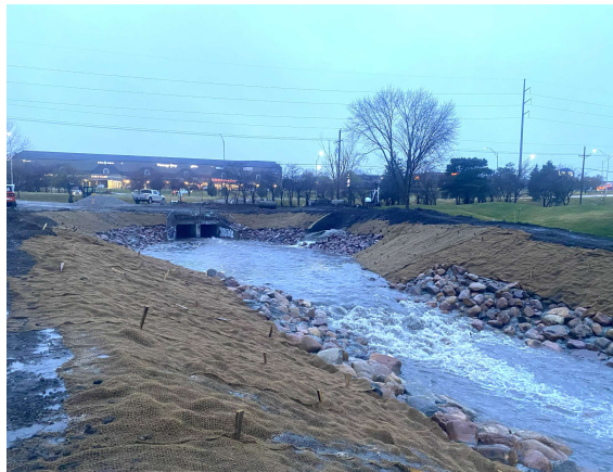
After: Restored channel and stabilized outfall (post-construction)
