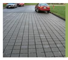
Permeable pavement is a GI practice that utilizes multiple sublayers of pavement to capture, store and infiltrate stormwater runoff to subsoil. Permeable pavement is ideal for cold weather climates. Precipitation can drain to sublayers and expand, which prevents surface refreezing and icy roads.
