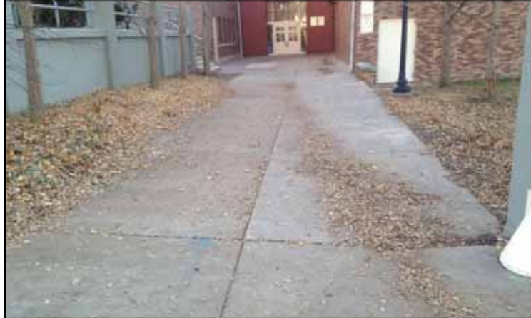
Driveway is very icy through winter due to water & north facing; runoff ends up in combined sewer
