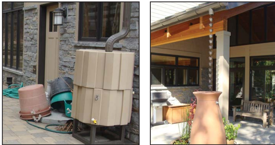
Figure 8-8 Examples of Residential Rain Barrels
