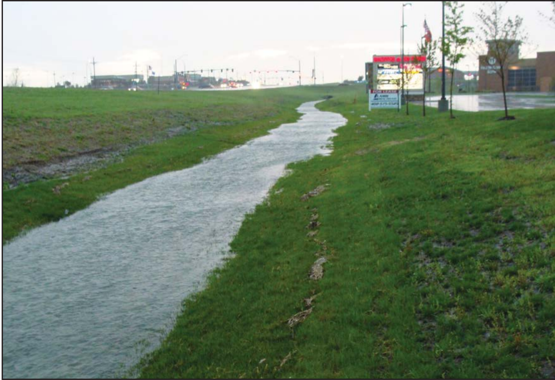
Figure 8-19 Bioswale
