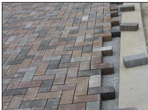
Figure 8-33 Example of a Permeable Paver Installation
