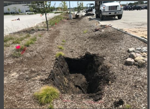
Excavated section of infiltration cell
