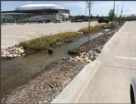
Water logged bioretention systems in northwest parking lot
