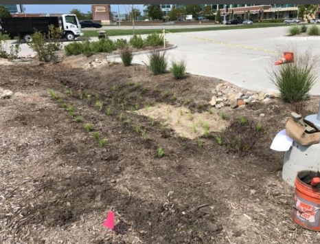
Palm and Fox sedge plugs and thin layer of mulch placed on top of repaired sections within the bioretention system
