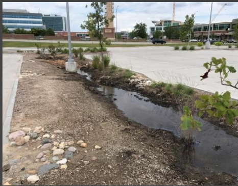
Water logged bioretention systems in northwest parking lot
