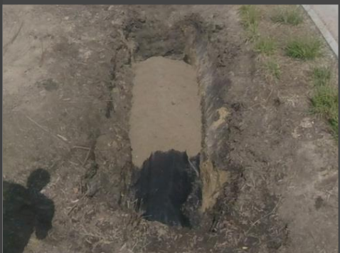
New 80/20, sand/compost BSM being installed
