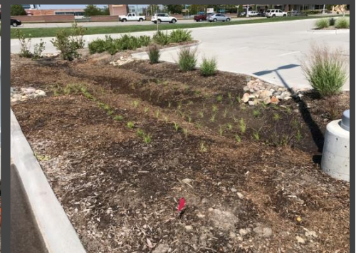
Palm and Fox sedge plugs and thin layer of mulch placed on top of repaired sections within the bioretention system
