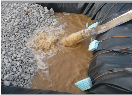
Construction dewatering operation with BMPs
