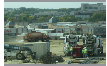
Water truck spraying water
