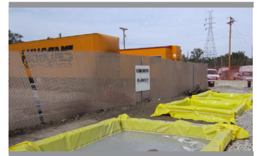
Concrete washout properly designated with secondary containment
