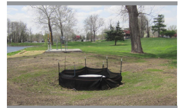
Construction inlet protection in good condition
