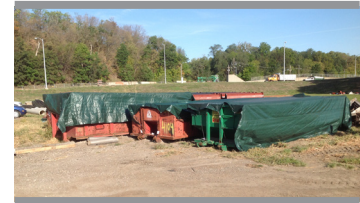
Appropriate waste management – covered dumpsters with labels (construction vs. municipal)
