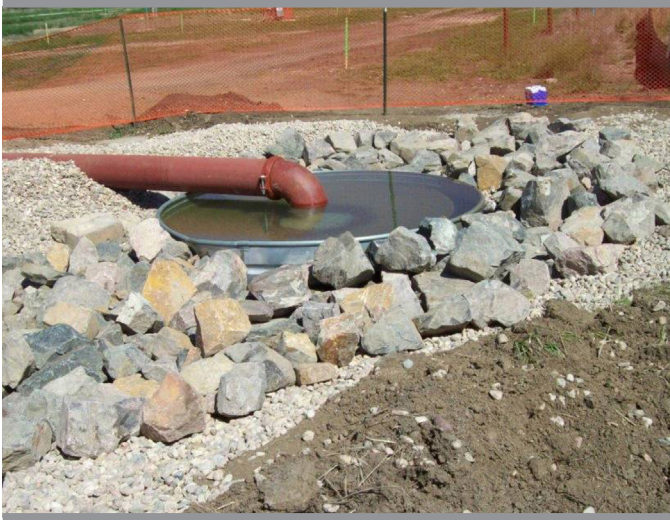
A stilling basin and energy dissipating rock outfall for a site discharging a large volume of construction dewatering water to a sensitive water
