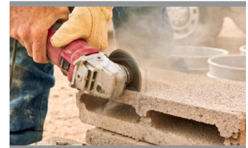
Construction workers using electric hand tools
