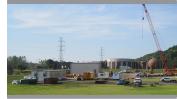
Well maintained Contractor staging
