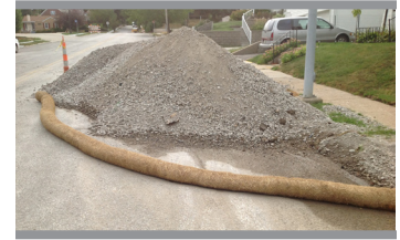
Gravel pile with BMP protection
