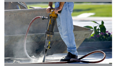
Construction with jackhammer
