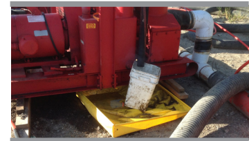
Drip pans provided for idle equipment
