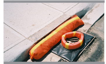
Construction with inlet protection in good condition
