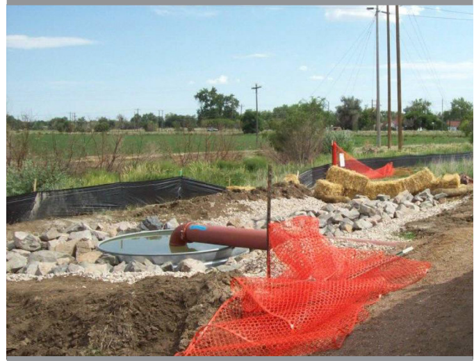
A stilling basin and energy dissipating rock outfall for a site discharging a large volume of construction dewatering water to a sensitive water
