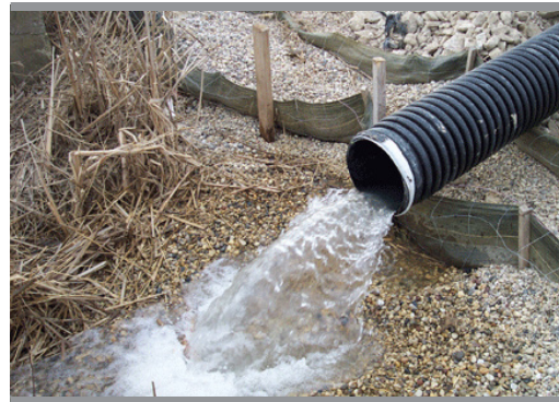
Dewatering discharge to approved offsite location
