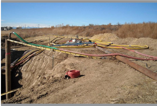
Dewatering system with wells and manifold for pipeline construction
