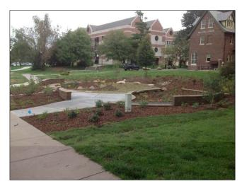
The two bioretention infiltration trenches
