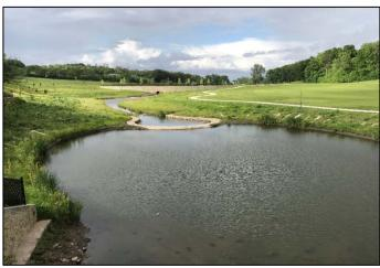
corner of the facility via two basin inlet pipes 72 and 84 inches in diameter. The basin outlet structure on the north east corner of the site controls the discharge of stormwater through two 48-inch basin outlet pipes into the downstream combined sewer system.
