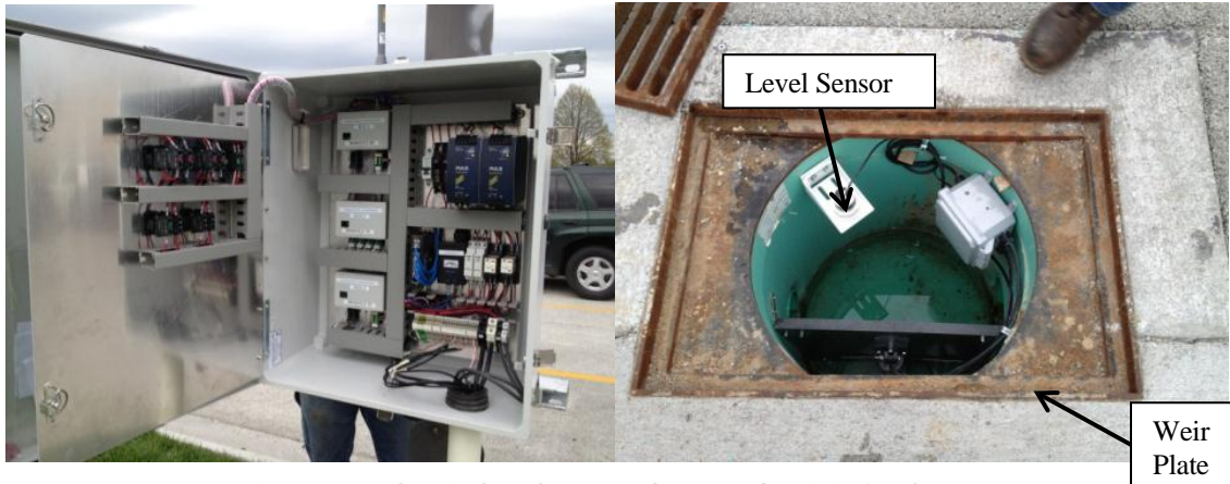
Figure 3-19. Electrical Enclosure and Actuated Weir in Omaha, NE.
