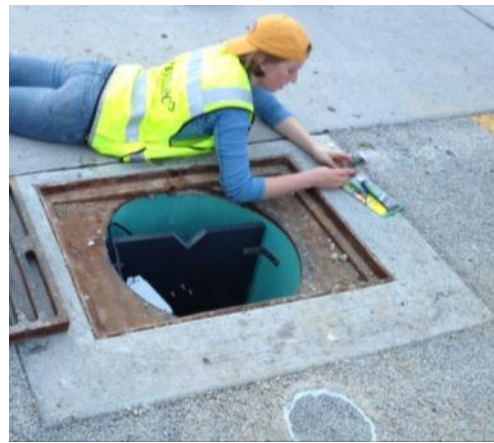
Figure 3-22. Personnel Placing Sealant Around Newly Installed Real-Time Controlled Weir Plate.
